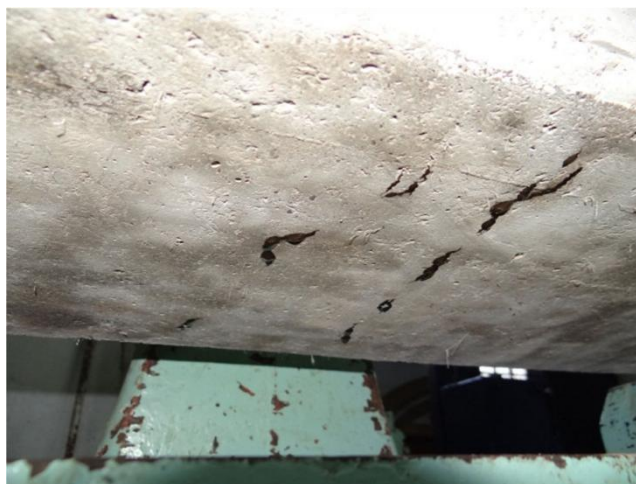
Soffit of slab after loading and crack formation Resin is released from voids through cracks Fig. 5
