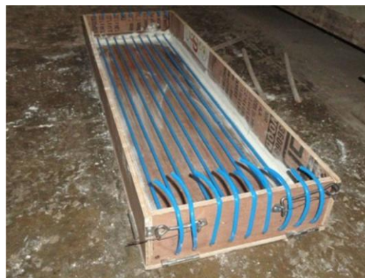
Arrangement of Void Former in Slab Fig. 2
